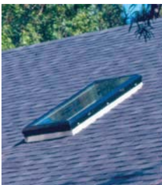
Use glass skylights; plastic will melt and allow embers into the home.
