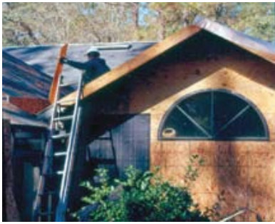
The roof is the most important element of the home. Use rated roofing material.
