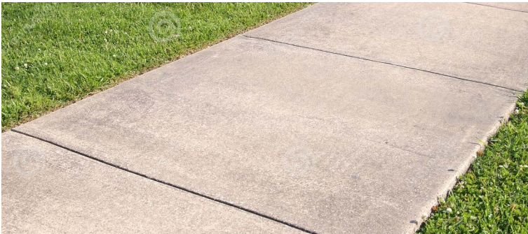
3. Concrete sidewalk as fire buffer and barrier
