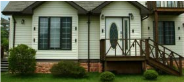
4. Stone wall skirt to protect the wooden wall body
