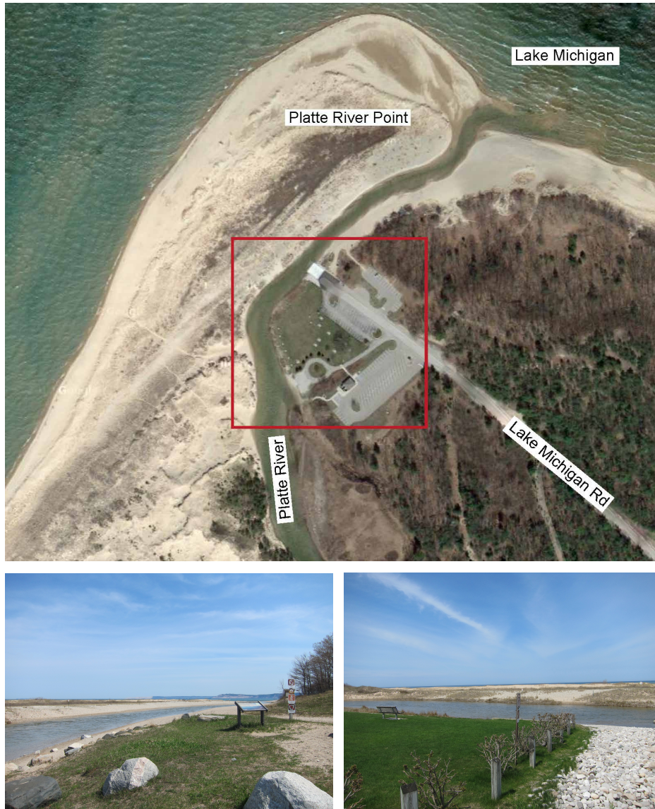
Figure 9. Platte River Launch Point
