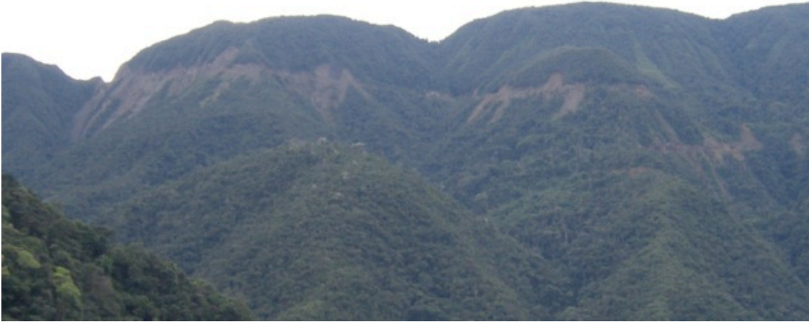
Figure 21: Landslides on the new road to Yokiri (Chapo Boyero-Otingamía)
