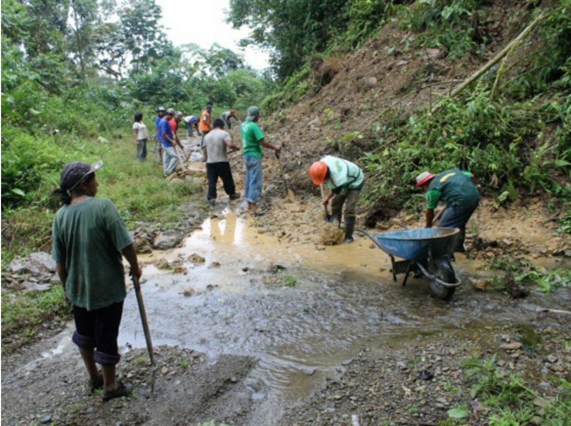
Figure 20: Yokiriños clear a landslide to open the road for Edison
