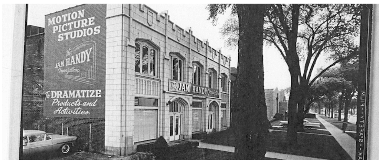
Exterior of the Jam Handy building, circa 1950s. Image from the Burton Historical Collection, Detroit Public Library
