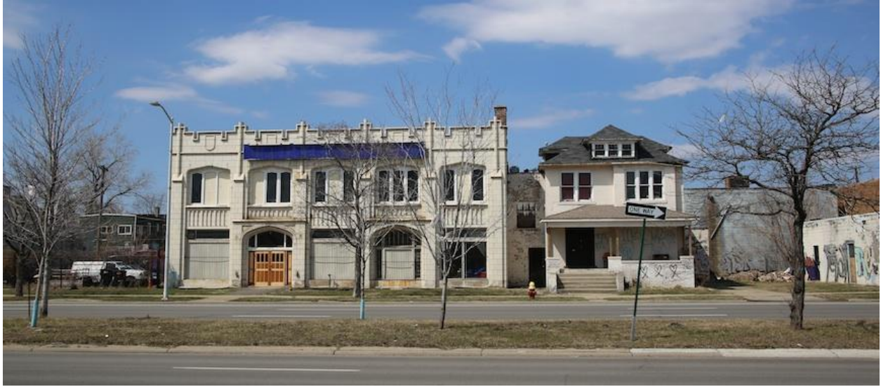
The Jam Handy Building, 2900 East Grand Boulevard, Detroit, Michigan. Photographed March 2014.
