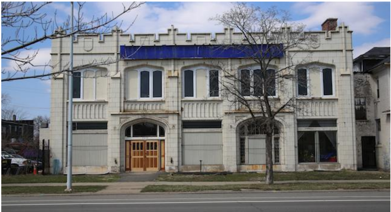
Top: View of East Grand Boulevard looking East. Photographed March 2014. Bottom: Façade of the Jam Handy Building.
