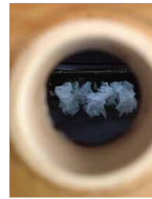
Uncoverd peephole looking into the structure from the outside
