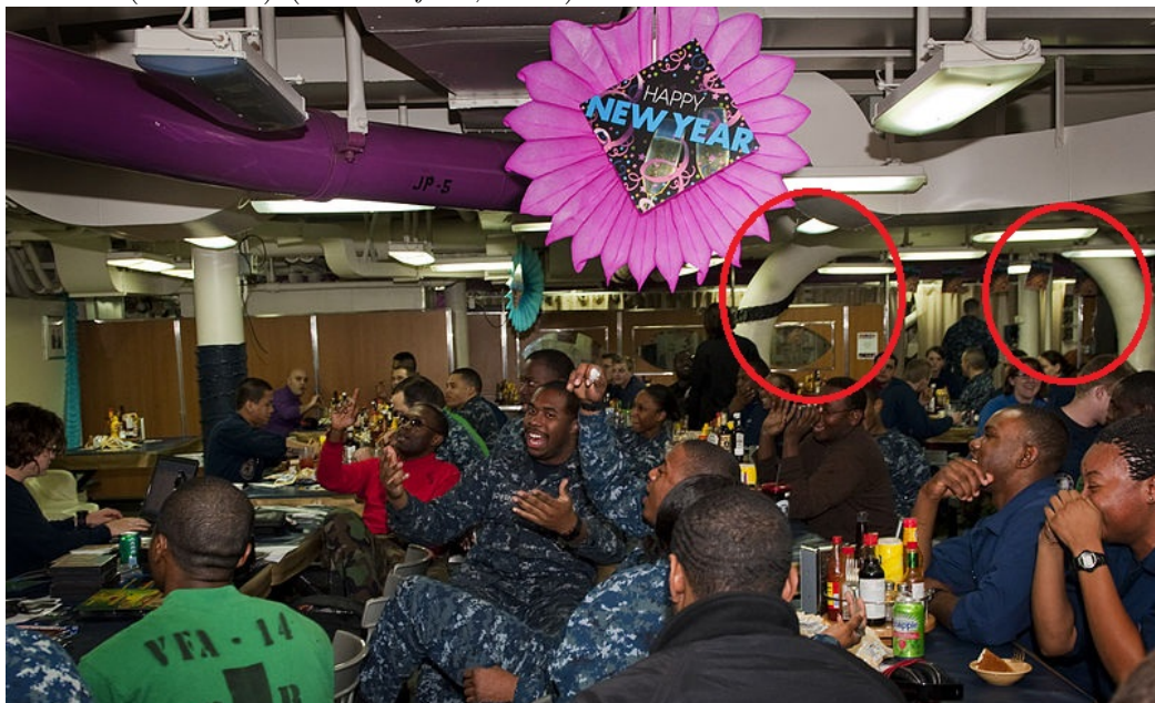
Figure 2.1: Example 1 of a sub-optimal distributed system layout. A jet fuel pipe, in purple, routed through the enlisted mess of the USS John C. Stennis (CVN-74) (Blumenfeld, 2012).
