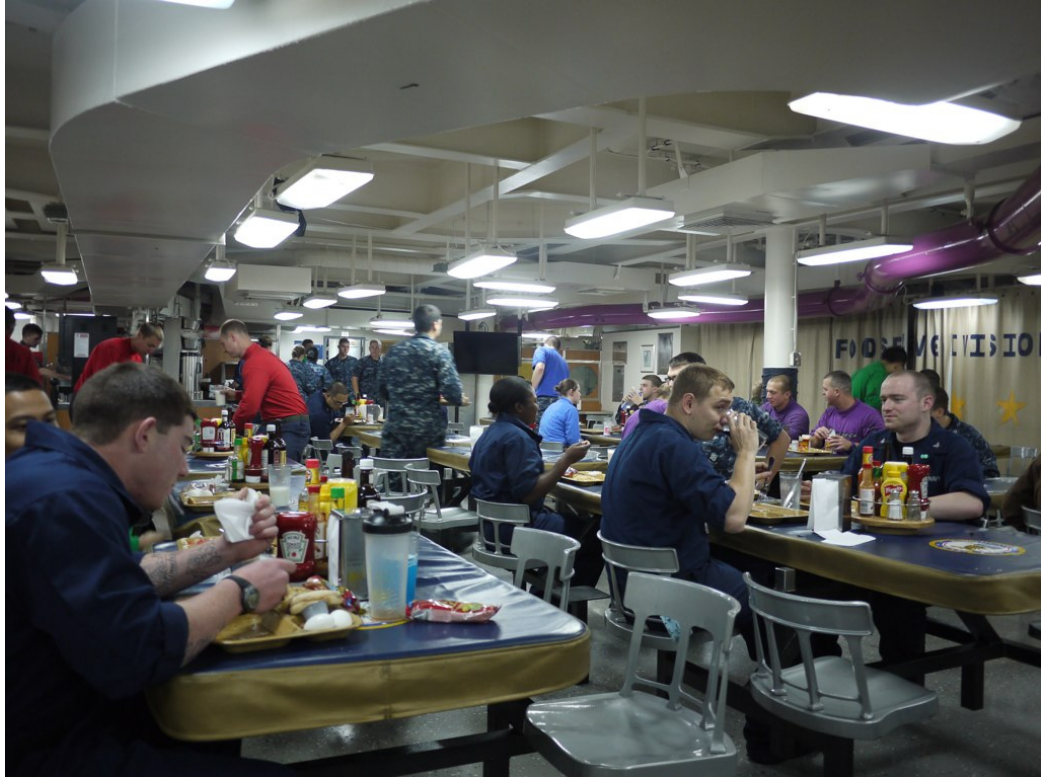
Figure 2.1: Example 1 of a sub-optimal distributed system layout. A jet fuel pipe, in purple, routed through the enlisted mess of the USS John C. Stennis (CVN-74) (Blumenfeld, 2012).
