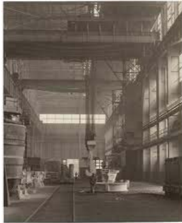
Figure 8: Ladle Hooks in Open Hearth Building
