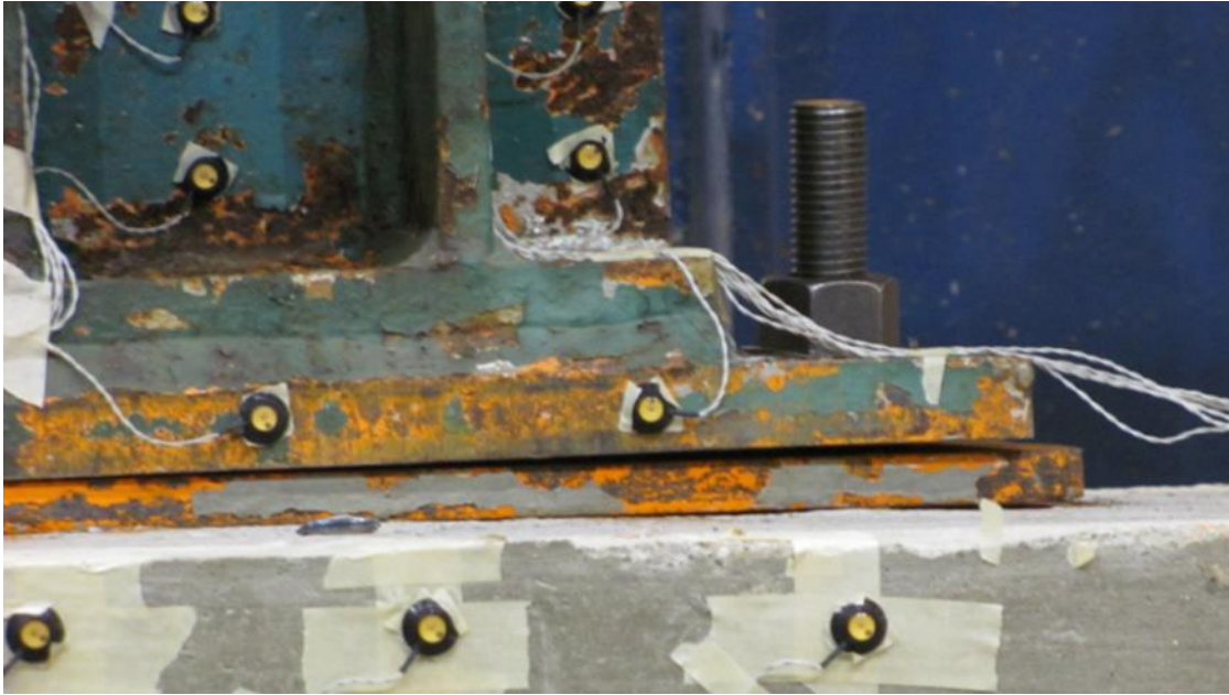
Figure 6.88 Photograph showing the rocking deformation mode of the bolster bearing
