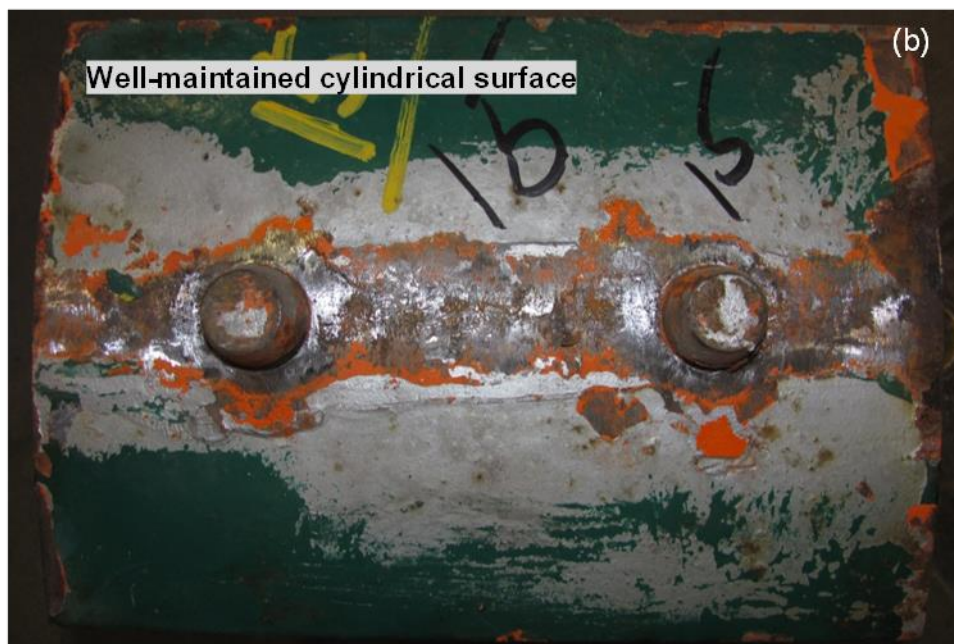
Figure 6.79 Pier bolster bearing #15 (PB15) in the as-received condition
