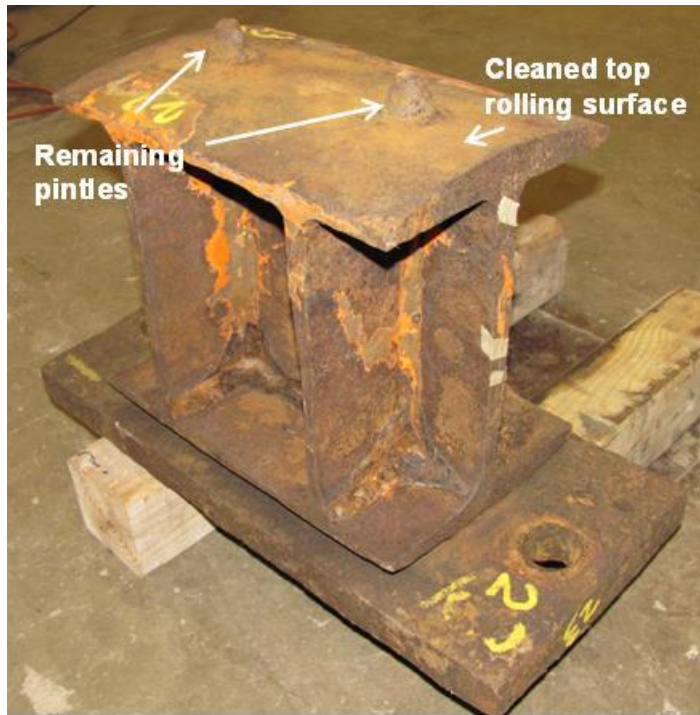
Figure 6.56 Bearing AR23 in its cleaned condition with rust removed
