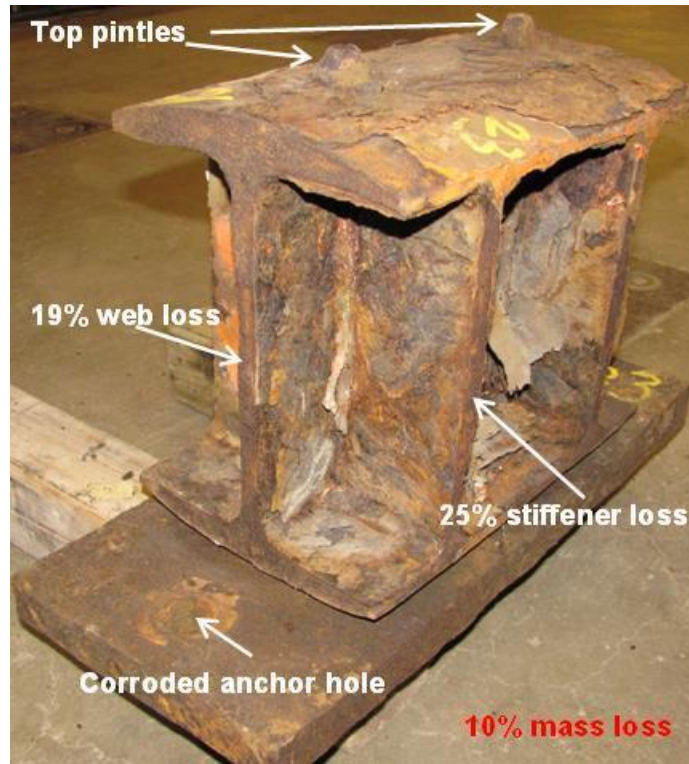
Figure 6.53 Abutment rocker bearing #23 (AR23) in the as-received condition
