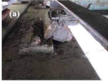
Figure 1.3 Toppled rocker bearing failures: (a) Birmingham Bridge (Splitstone et al. 2010) and (b) Dunn Memorial Bridge (NYSDOT 2005)
