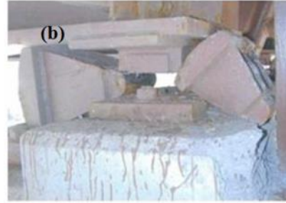
Figure 1.3 Toppled rocker bearing failures: (a) Birmingham Bridge (Splitstone et al. 2010) and (b) Dunn Memorial Bridge (NYSDOT 2005)
