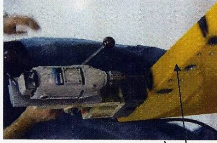
Horizontal bolt holes were not machined onto lift platform
