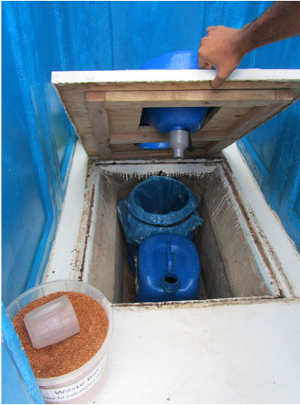
Figure 4. Image of inside of Sanergy toilet showing the separate containers.
