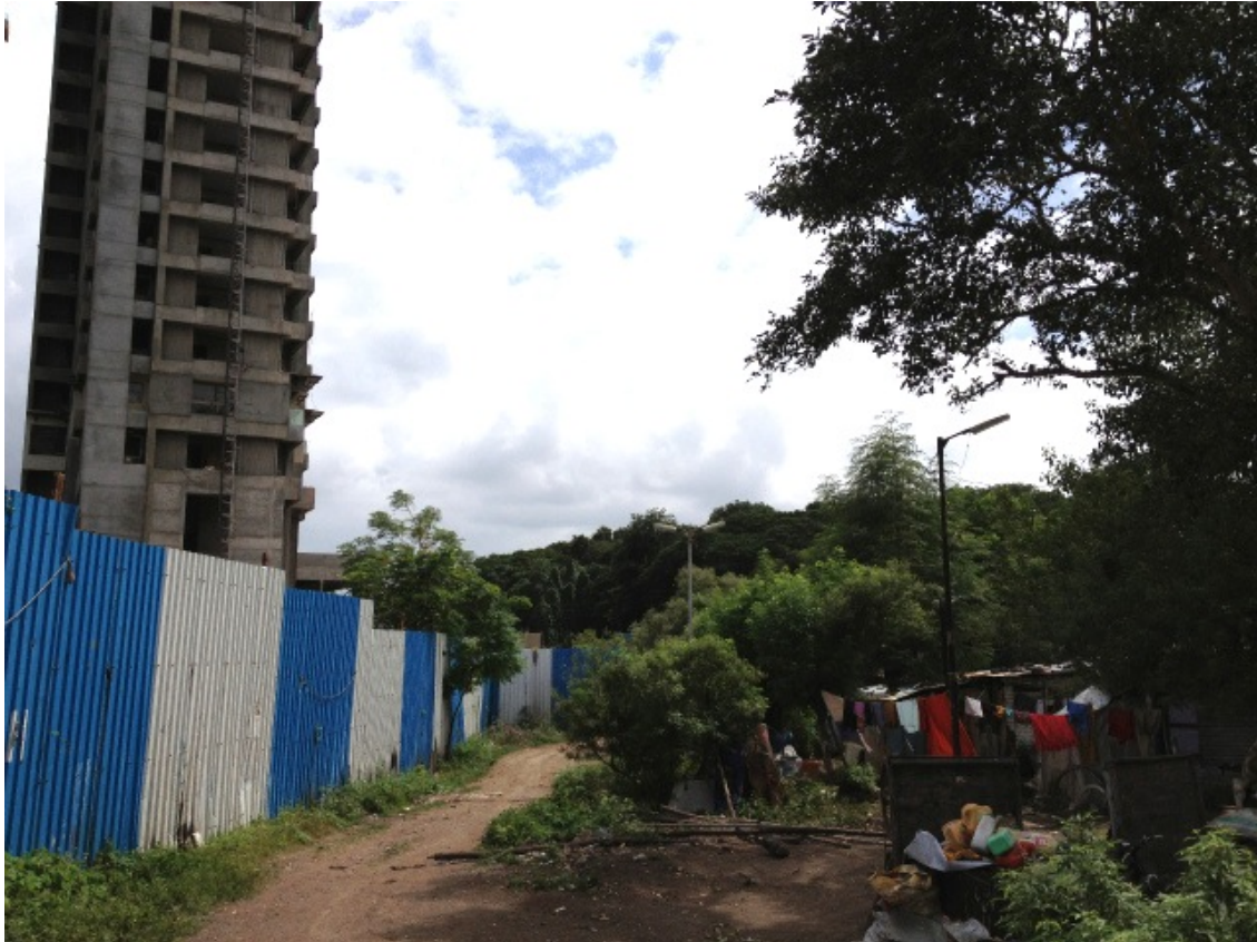
Figure 5.2 A slum in dispute with the military authority in Pune
