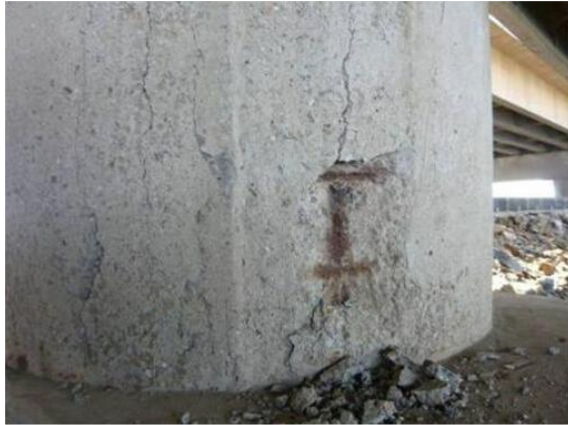
(a) Bridge column
