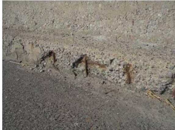
(b) Bottom of the bridge wall
