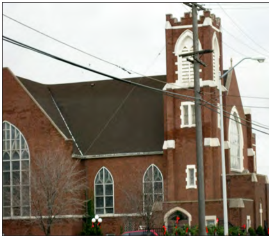
Figure 2.1. Trinity St. Mark's Church on Fort Street
