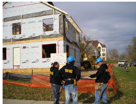
Figure 6.2: Christian Center Home Repair Project, Milwaukee, WI Source: www.mccwi.org
