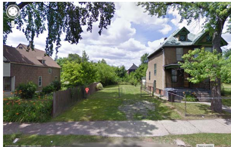
A house with an adjacent cared-for lot that faced prospect of Hantz purchase in February 2013. Google Images, 2013.
