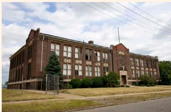
Figure 2.19. The Breitmeyer School on Cameron Street is demolished.
