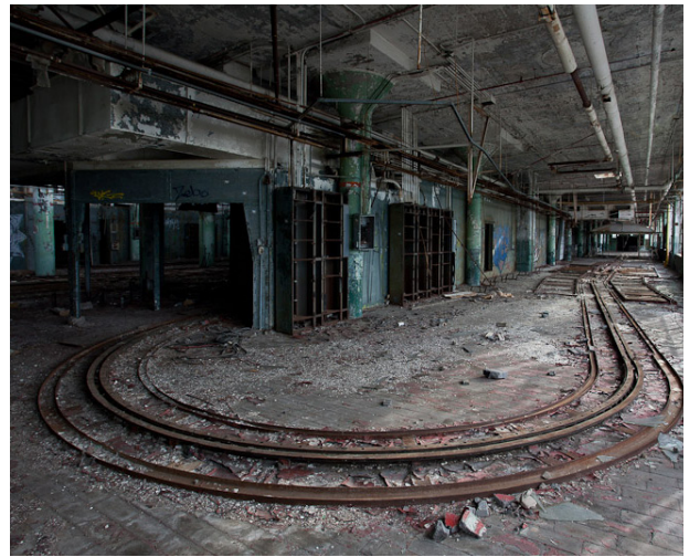
Figure 7.33. Production line on top floor of Fisher Body Plant No. 21.
