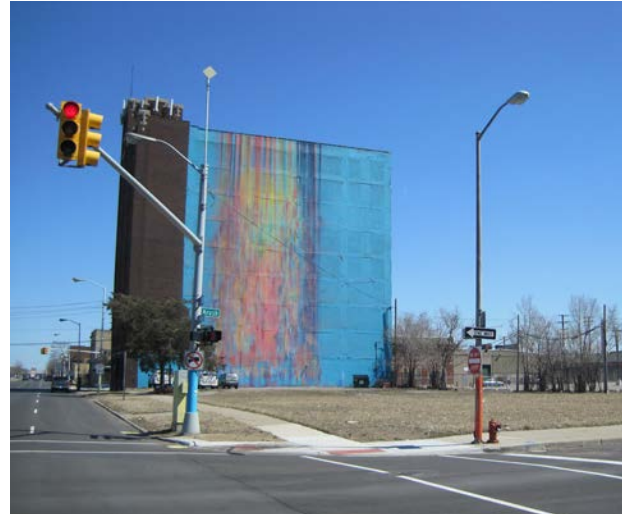
Figure 7.15. Existing conditions at potential Illuminated Park.
