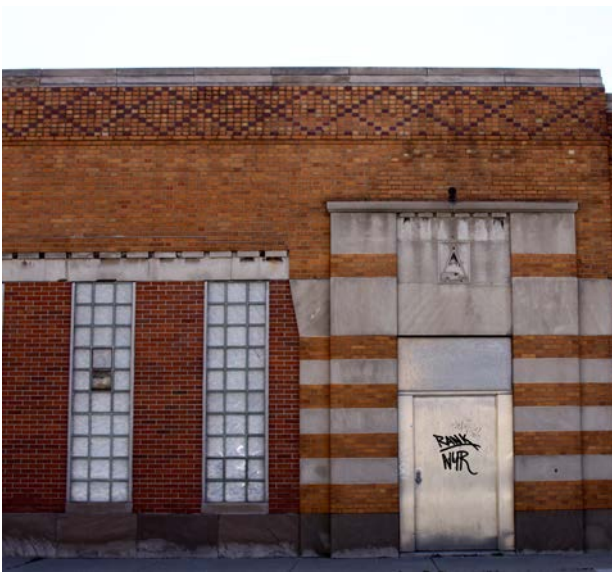
Figure 7.4. The former Autocar Sales building at 290 Piquette St. is an example of the Art Deco style.
