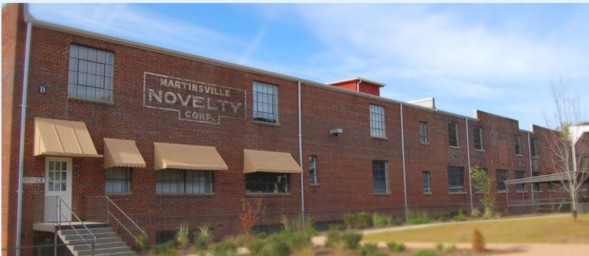
Figure 6.4. The Martinsville Lofts project.
