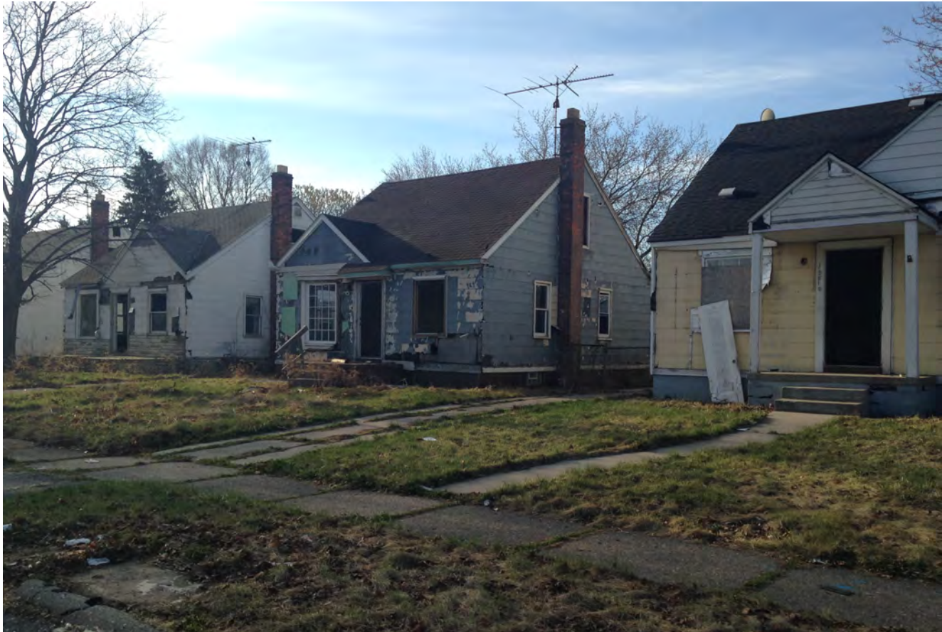
FIGURE 4.1 | Vacant, open, and dangerous houses on Liberal St.
