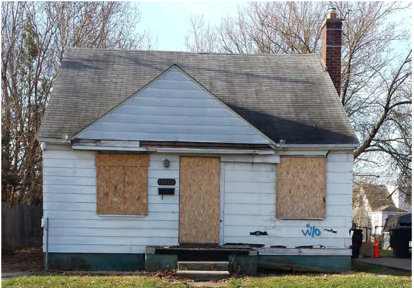
FIGURE 4.4 | Boarded-up house on Liberal St.
