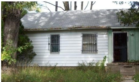
FIGURE 3 TYPICAL HOME WITH POOR EXTERIOR AND LAWN MAINTENANCE.
