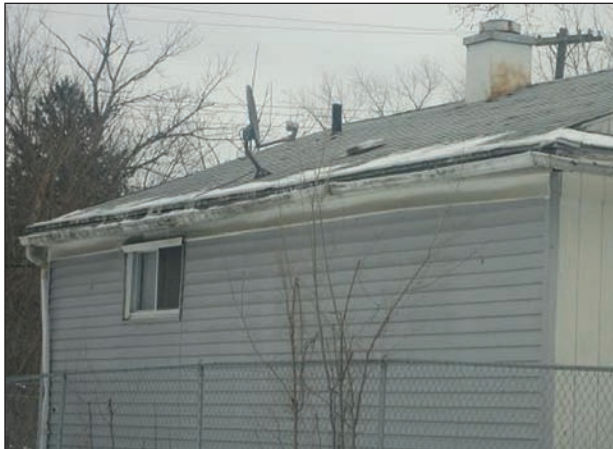
Figure 5.8: Gutter Repair Needed
