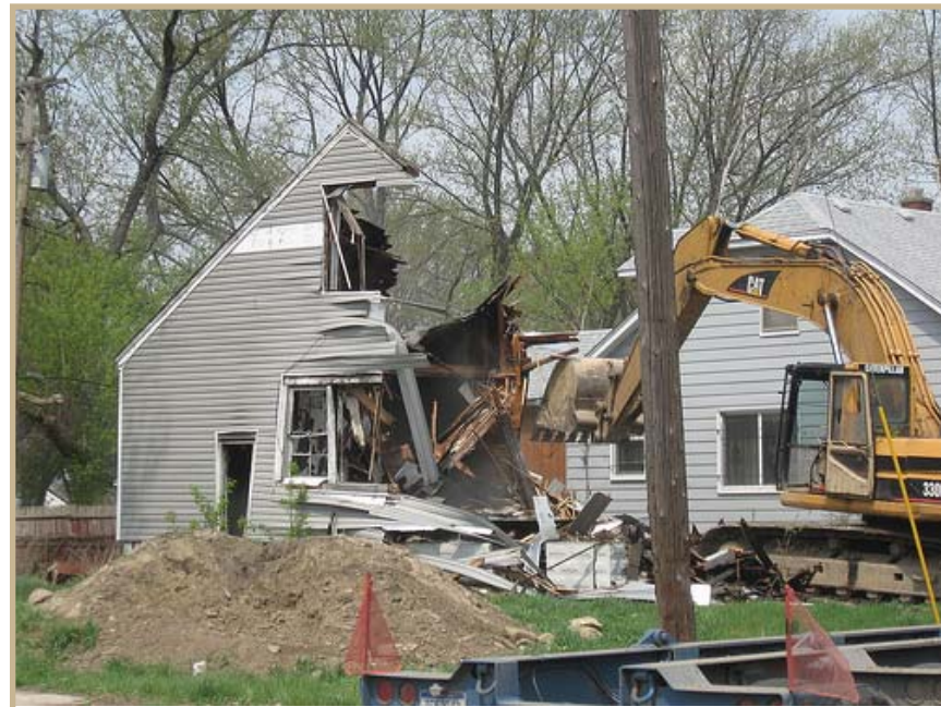
Figure 6.7: A house being demolished
