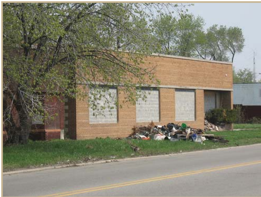
Figure 9.9: Dumping in front of a vacant building on Schoolcraft Road
