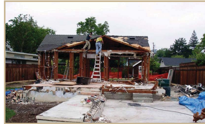
Figure 4.8: House in the process of being deconstructed
