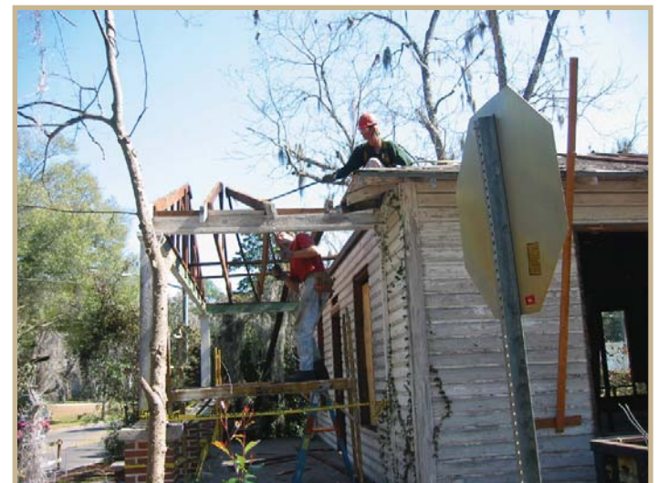
Figure 6.8: A derelict house being deconstructed
