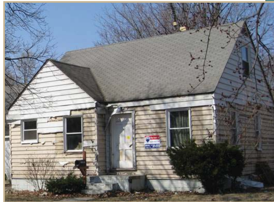
Figure 6.4: A house with code violations
