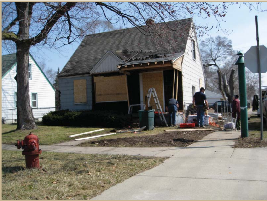
Figure 6.9: A house being rehabilitated
