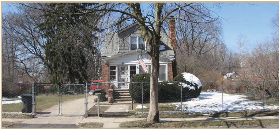
Figure 7.6: An existing Detroit homestead in Brightmoor that includes a house and fenced-in vacant lots on both sides
