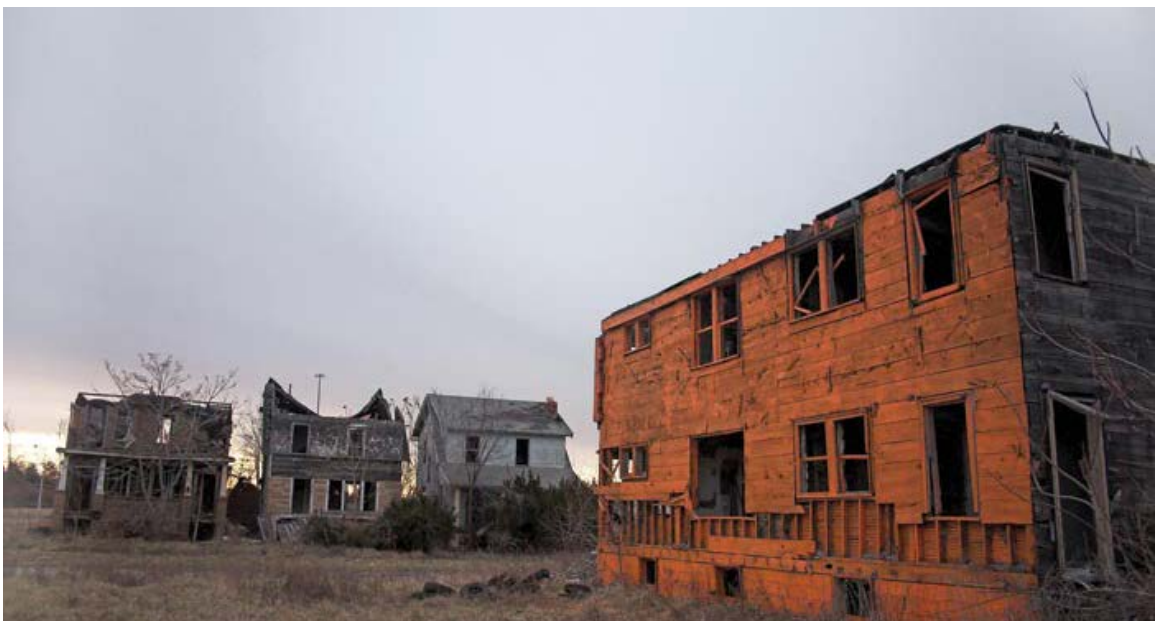
[Figure 17 + 18] Detroit Demolition Disneyland, 2005-2006 Source: The Unreal Estate Guide to Detroit , Andrew Herscher
