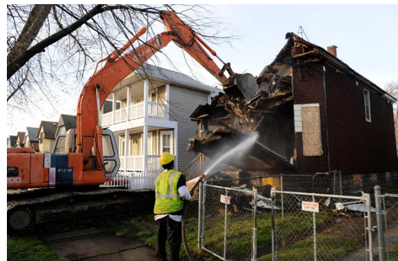
[Figure 05] Lead dust mitigation through water hosing Source: Associated Press
