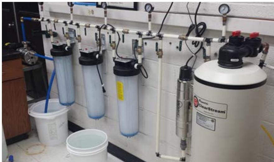
**Figure 7.** The purification system was designed by the LBC team before the semester. It contains a pump, three cartridge filters, a UV bulb, and an activated carbon tank. The control system will have to interface and communicate with the pump at the front end of the system in order to prevent the purification system from running dry.
