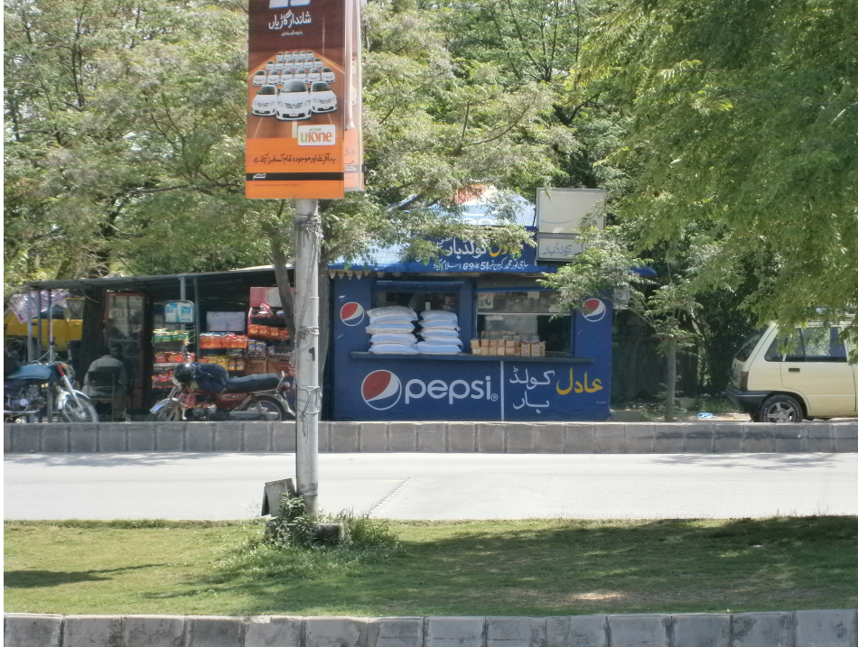
Figure 14. Photo of a licensed kiosk in Islamabad using durable construction material following the prescribed design set by CDA. The shed to one side is an illegal extension, using semi-permanent materials and construction techniques.
