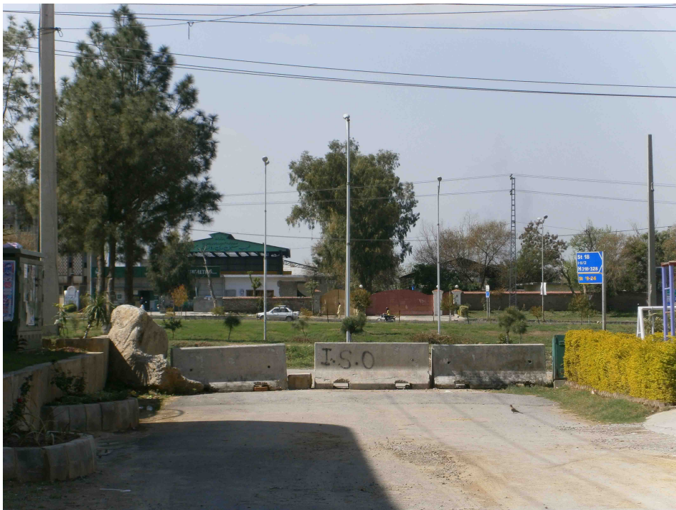
Figure 83. Blocking off of a through road in the subsector I-8/2 using concrete blocks
