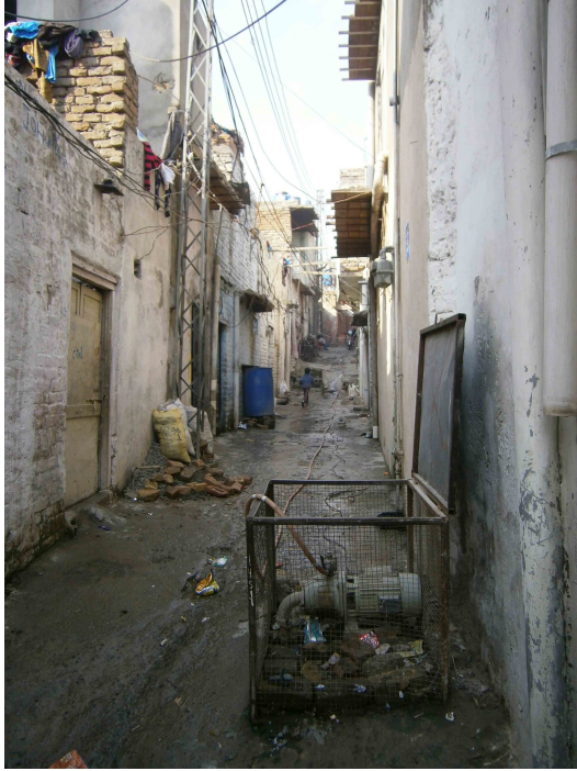
Figure 57. Shared tube-well
