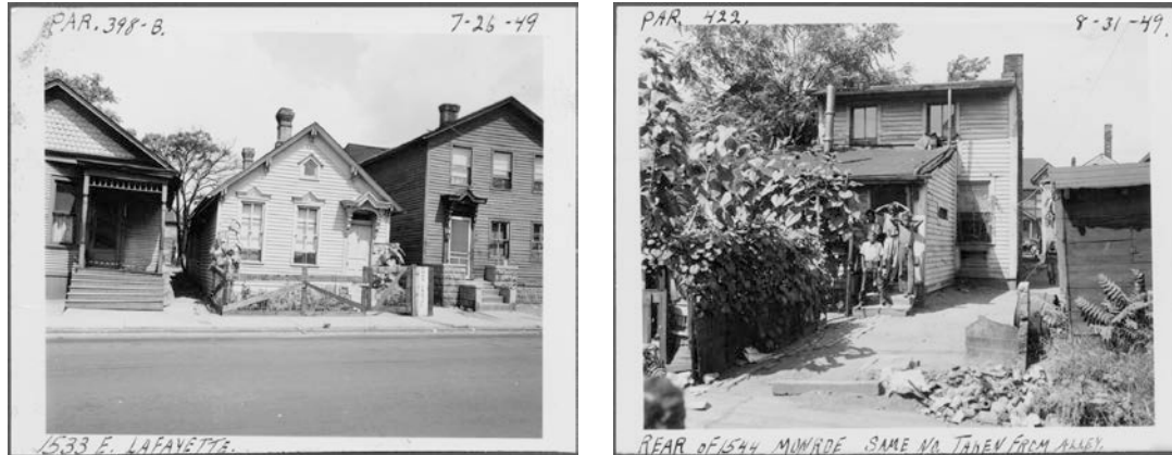
Figures 2.13 and 2.14: Although photographed in 1949, these images of Black Bottom suggest some of the ways Detroit's African American Migrants of the early twentieth century made use of their yards and this housing stock for gardens. On the left, sunflowers and other plants grow in a fenced area in front of a Victorian-era cottage. On the right, sunflowers and beans grow in the rear of a home. These images, and hundreds more, were taken by photographers for the Detroit Corporation Counsel, the agency vested with documenting and appraising the value of the neighborhood before it was razed to make way for Interstate 75. Corporation Counsel – Real Estate Division Records, Burton Historical Collection, Detroit Public Library.
