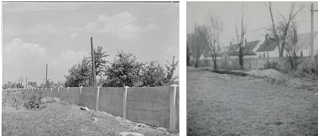
Figure 2.19: Concrete Wall, John Vachon, 1941. Library of Congress, Prints and Photographs Division, FSA/OWI Collection, LC-USF34- 063680-D. Figure 2.20: Concrete Wall c. 1974. Burniece Avery Papers, Detroit Public Library.
