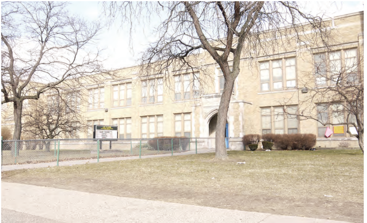
Figure 2.13: John Clark elementary school
