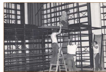
Construction of the 'stacks' of the Bentley.
