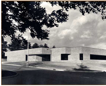
The new home of the Michigan Historical Collections, the Bentley Historical Library.
