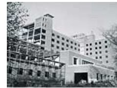
South Quad Dorm under construction, May 1952
