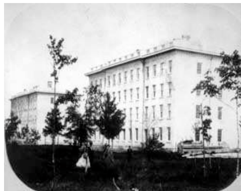
Mason Hall, 1861 Original University Instructional Building in Ann Arbor, built in 1841
