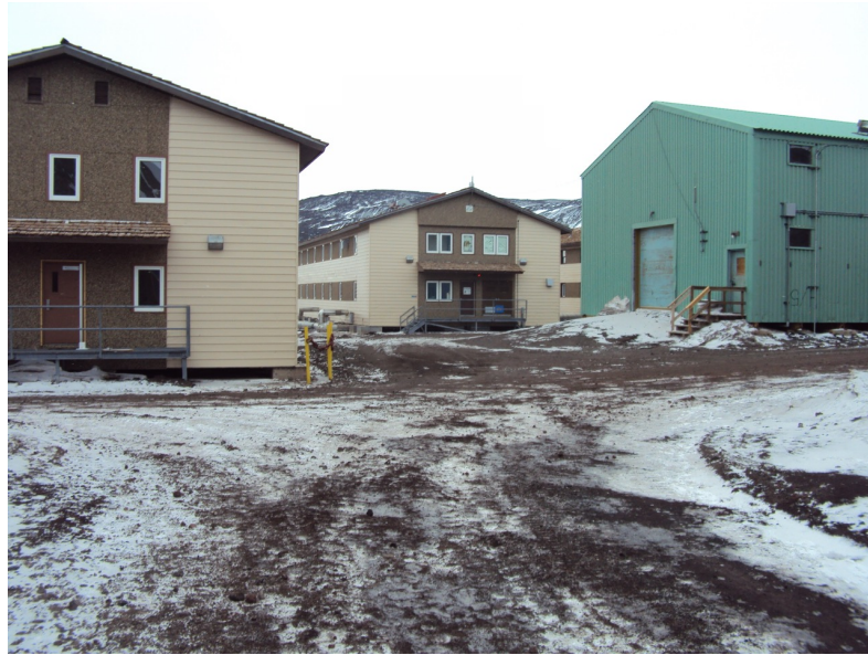
Figure 5.100: View of the dorm buildings in McMurdo where we spent the ‘nights’. We were two to a room. Bathrooms were shared and we were encouraged not to shower every day to save clean water. Each building also had laundry facilities (each room was assigned one laundry day per week) and common living areas with seating, board games and televisions.
