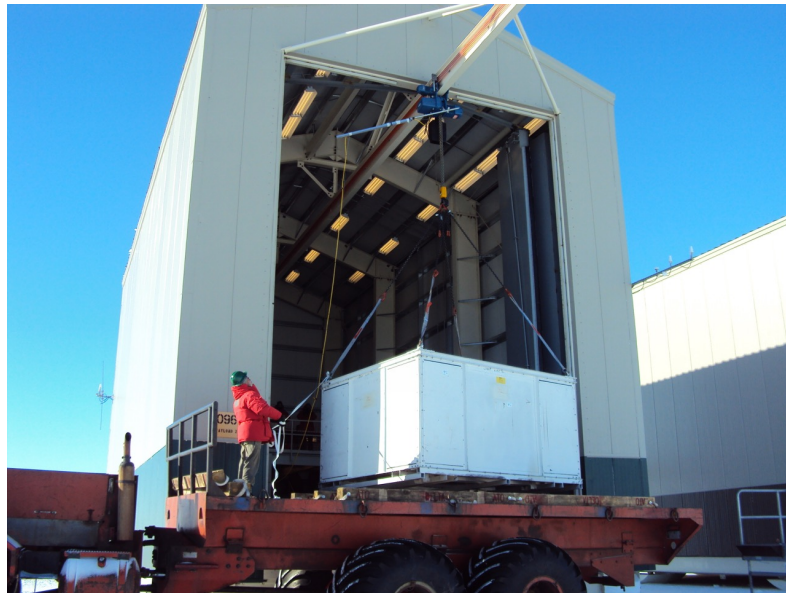
Figure 5.51: Lifting CREST into Hangar 096 via sliding ceiling crane.
