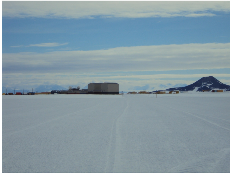
Figure 5.98: View of LDB from the launch pad. All non-tent buildings are deployed on skis and moved to higher ground every winter. Otherwise, non-mobile buildings eventually sink below the ice surface.
