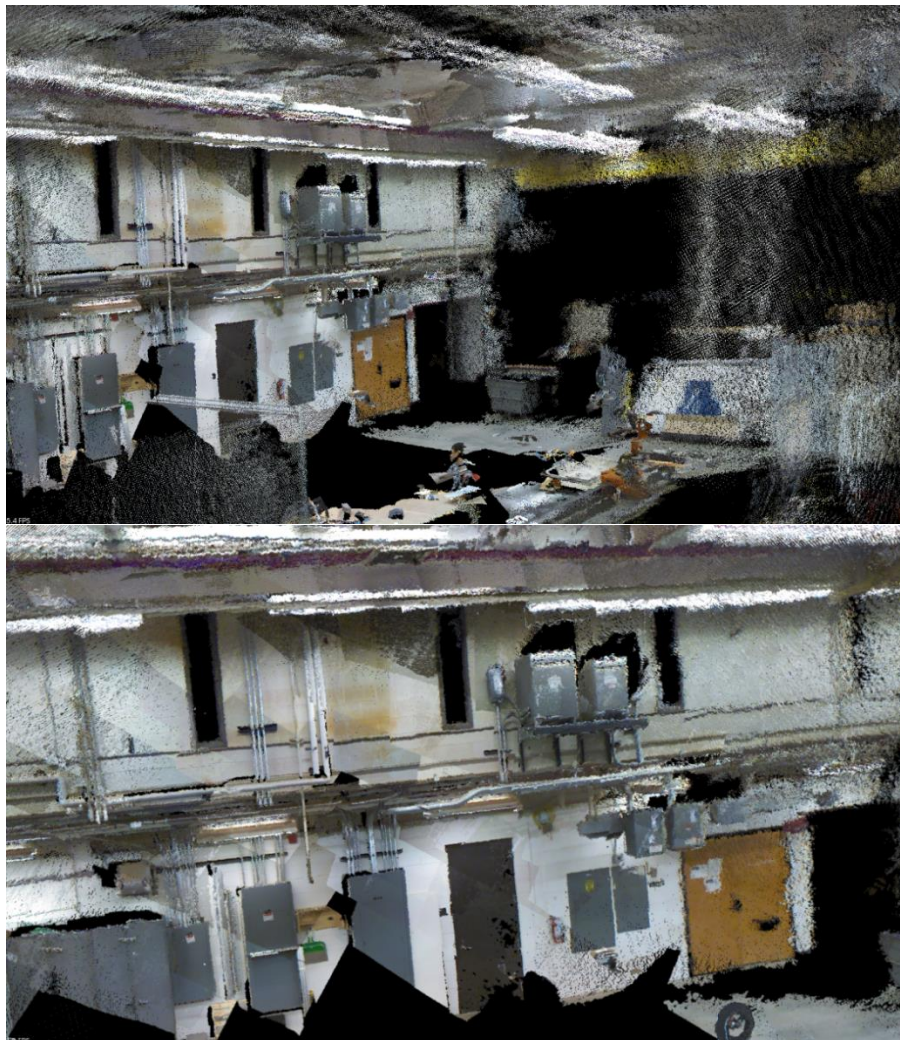
Figure 5-9: An as-built 3D point cloud of the FabLab at the University of Michigan
