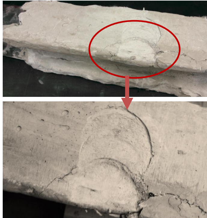
Fig.2.14 Damage condition of FR-ECC protected steel beam after eccentric impact
