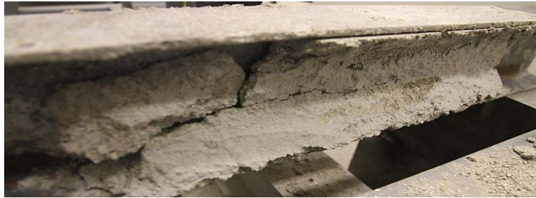
(e) After 4 th series of impacts (cracking and delamination of SFRM on web)
