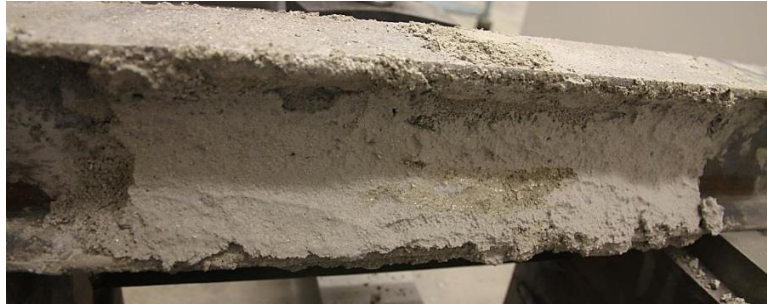
(d) After 3 rd series of impacts (complete delamination on top flange)
