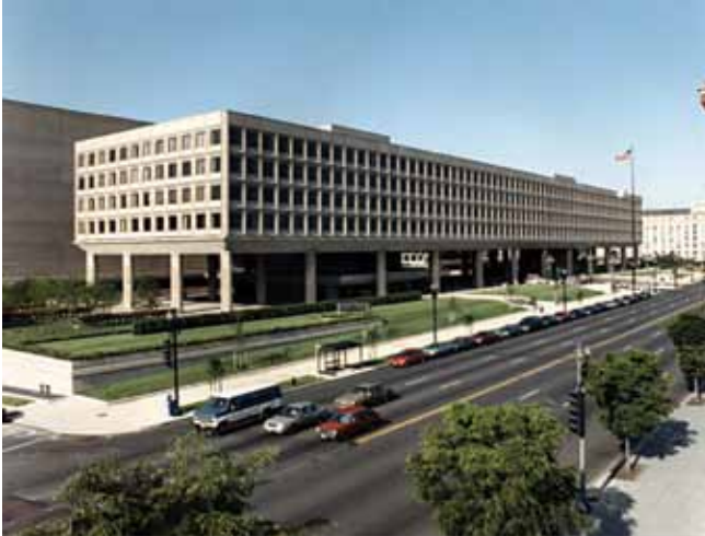
U.S. Department of Energy Headquarters
