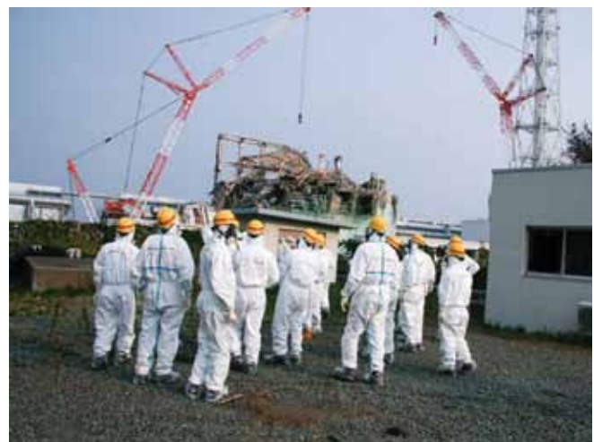
The emergency cooling generators were flooded leading to hydrogen explosions in the plant.
