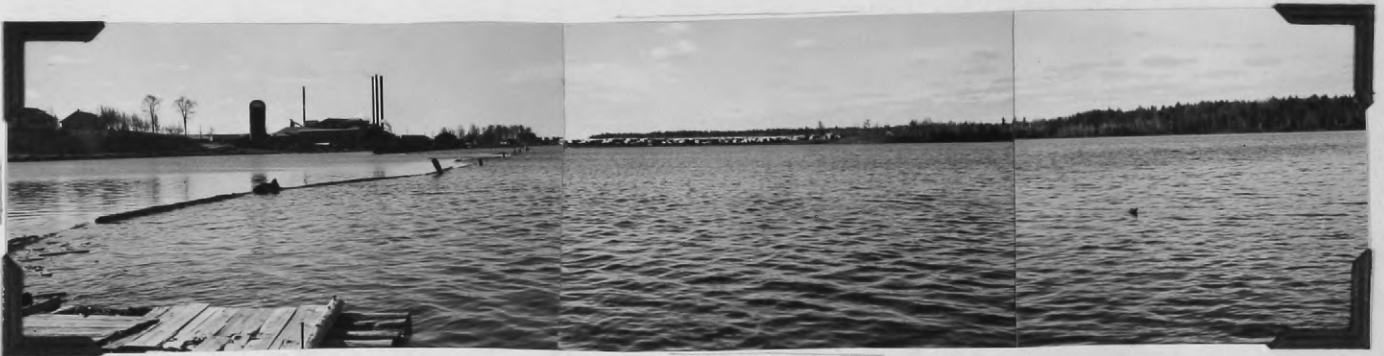
PLATE I. Typical Lake States Lumber Mill Showing Yards and Timber Supply
