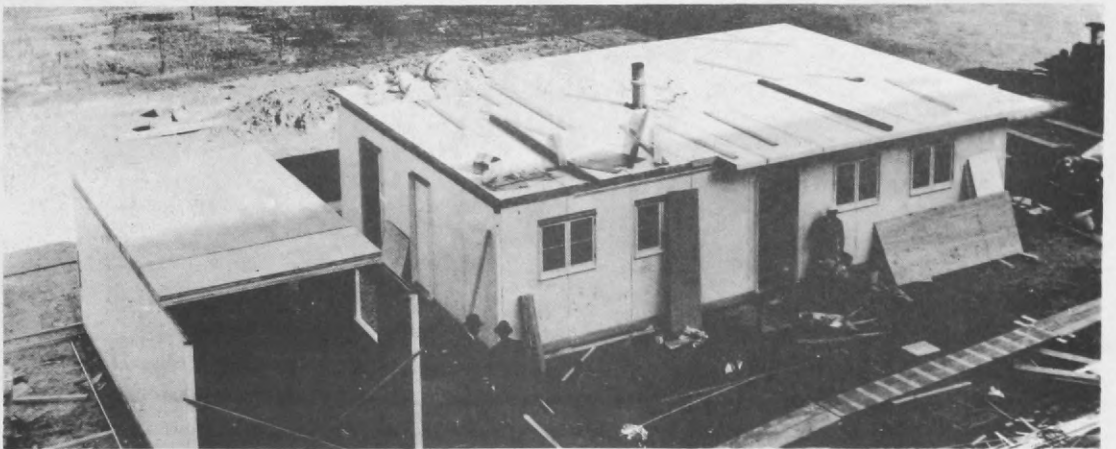
All house panels assembled and garage nearing completion
