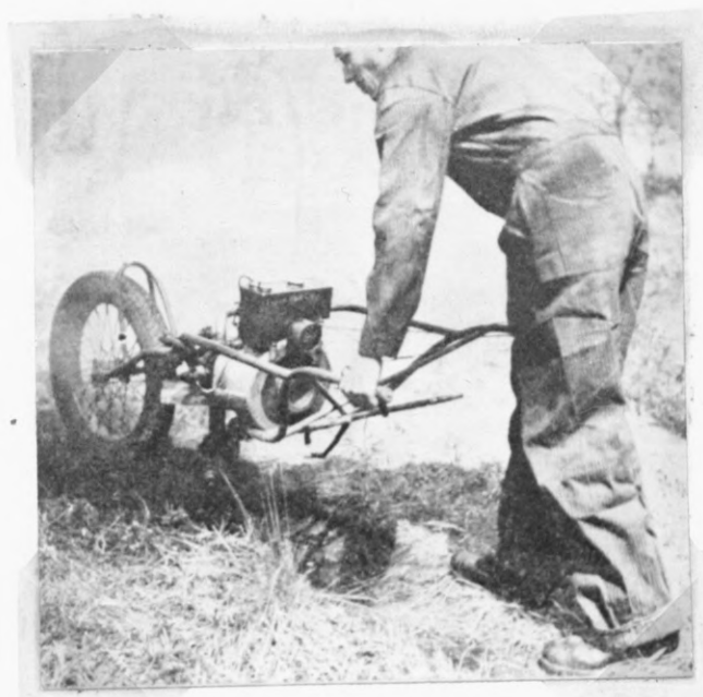
Fig. 8. Bosworth trencher. (After a photo by the U. S. Forest Service).
