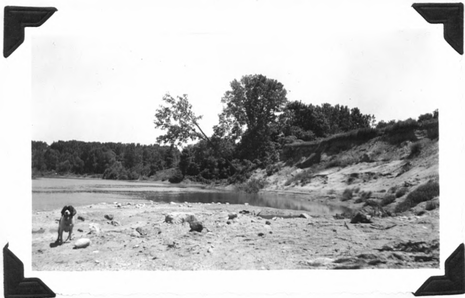
Bank Erosion 1 mile below Oxbow Farm. In the April, 1937, flood, the Thames gouged 5 acres out of a cropland at this point.
