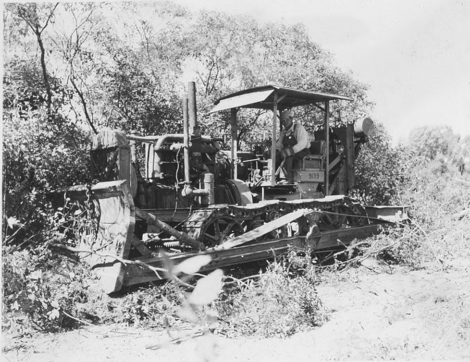
Clearing with a bulldozer
