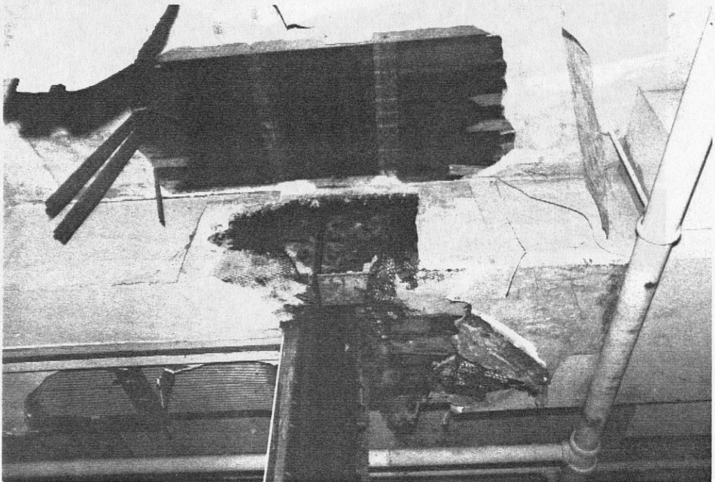
Fig. 6.13 Details of Steel Frame in Building G
