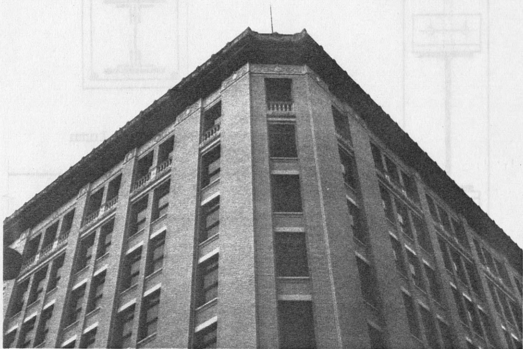
Fig. 6.20 Parapet of Building J
