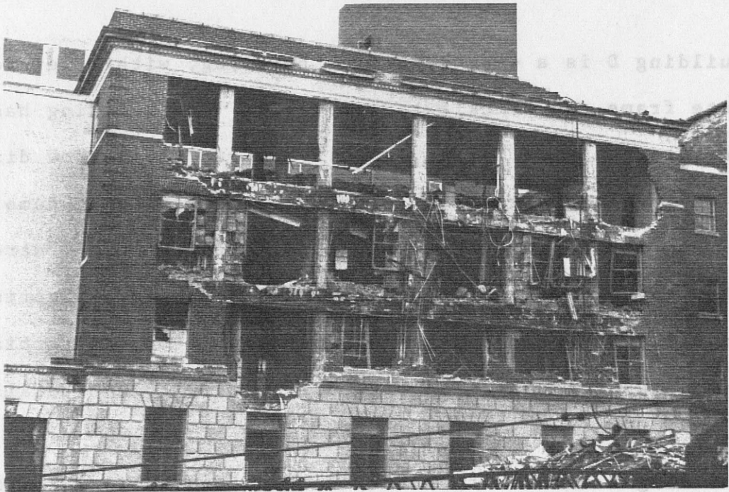
Fig. 6.7 Building D During Demolition
