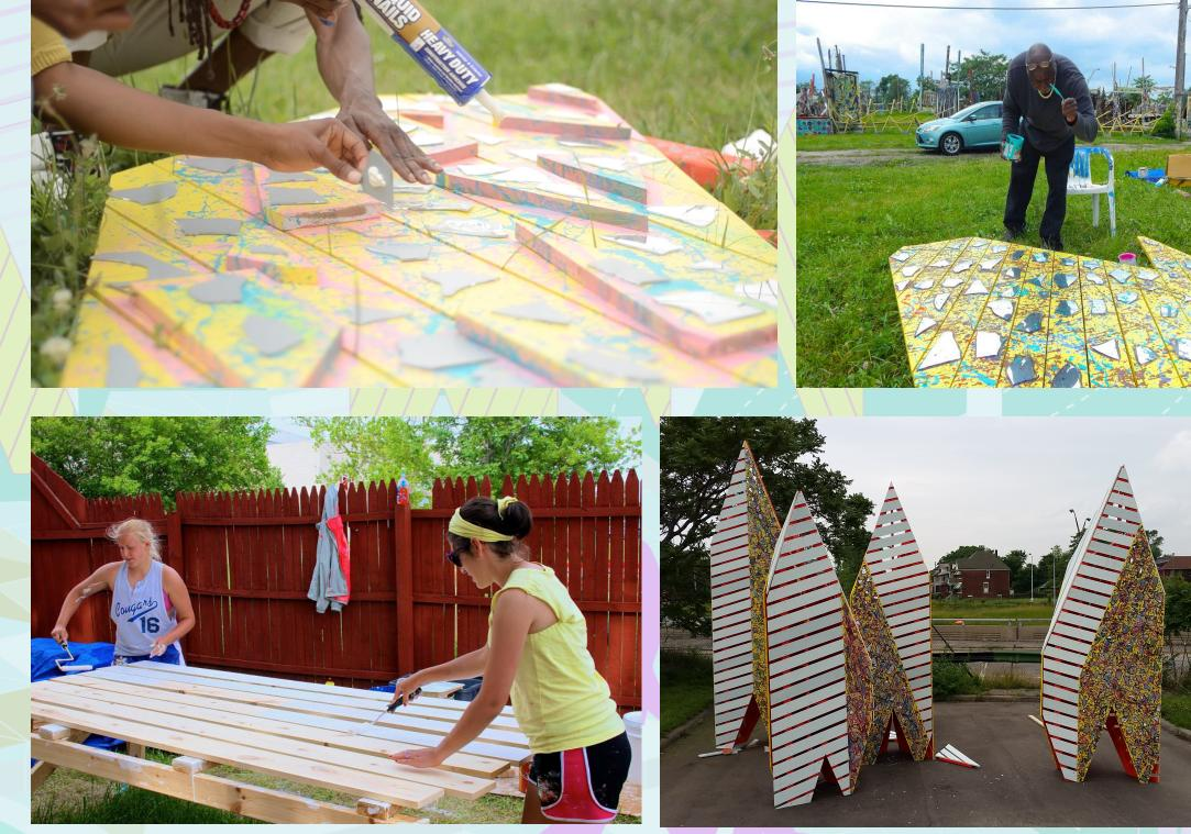
After being primed, the framing was constructed with two layers of pinewood 2x4's with plywood gussets in between, secured with liquid nails and screws. Plywood cladding was then primed and painted before screwing them into the framing. After, Dabls saturated select boards with his art. The mirrors and small wood pieces that were used by Dabls was put on with liquid nails and screws.
