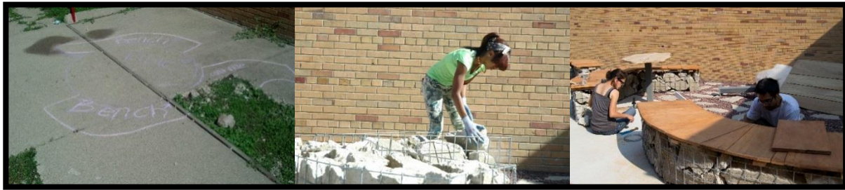
Fig. 5-4 Building gabion benches
