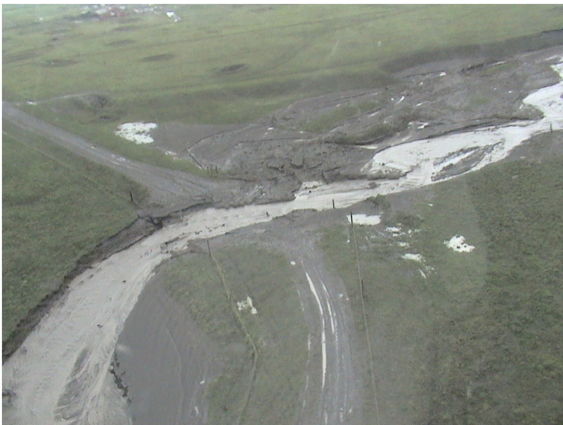
Figure 20: A lahar from the July-August 2008 eruption washed away a bridge on the Umak Island. Photo taken July 24, 2008 by Lonnie Kennedy of the Alaska Volcano Observatory, University of Alaska Fairbanks
