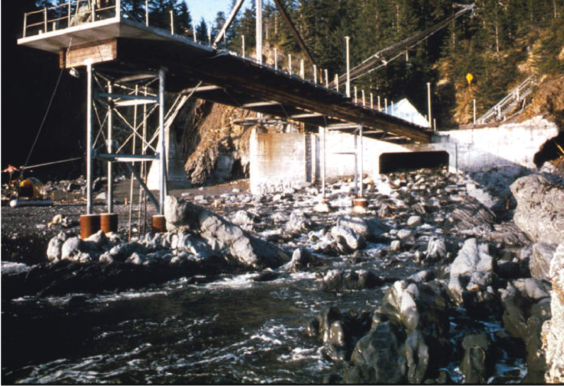
Figure 4: Photo showing the uplift of a dock on Hinchinbrook Island near Prince William Sound. The dock and surrounding land was uplifted by nearly 2.5 m during the earthquake. Photo by J.K. McGregor and C. Abston, USGS.
