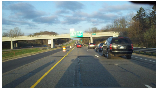
Figure 2 - New Construction on M-14
