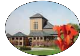
Lurie Engineering Center
