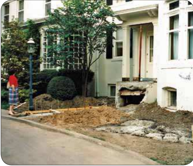
Preparations for a handicap ramp
