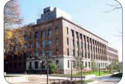
East Engineering Building
