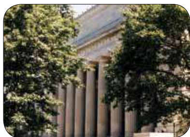
Angell Hall Renovation
