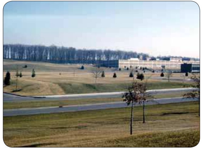
1970s Early construction on the North Campus
