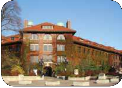
West Engineering Building
