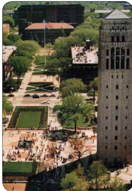
Ingalls Mall/Diag Re-construction
