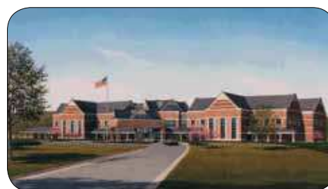
East Medical Complex Plymouth Road
