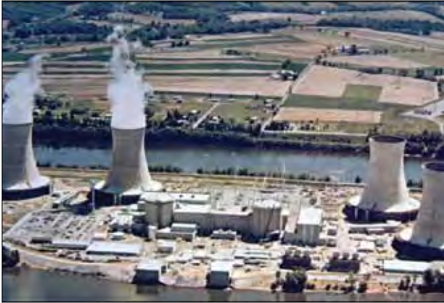
The Three Mile Island nuclear plant
