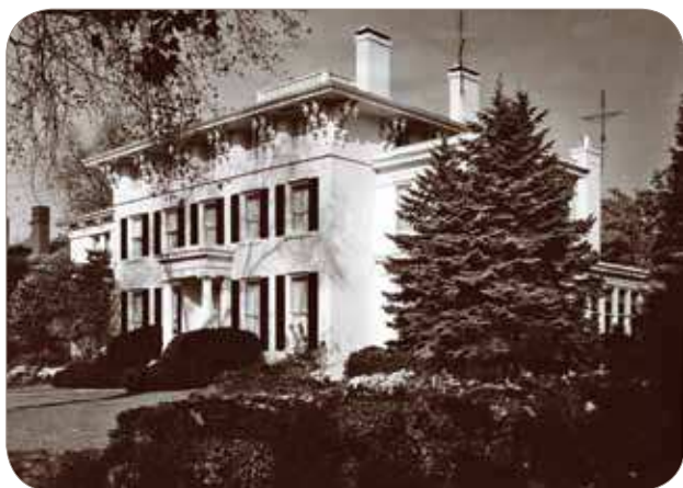
Mrs. Ruthven's Plant Room (right)
