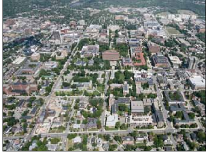
Aerial of the Central Campus
