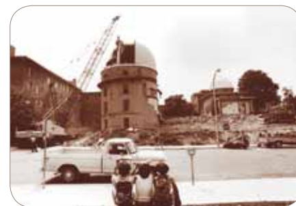
Demolition of the old Astronomy Building
