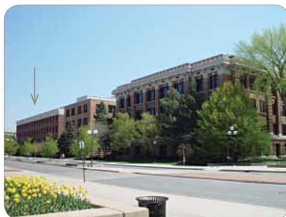
Chemistry Buildings - Dow Laboratory (left)
