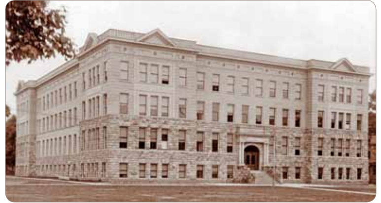
New Medical Building
