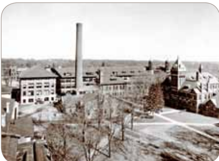
West Engineering, Engineering Shops Old Heating Plant
