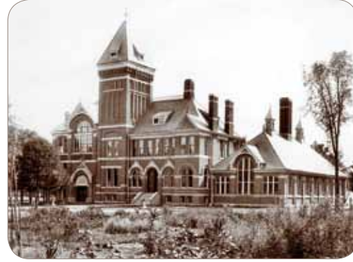
The Engineering Shops With the tower and forge (right)
