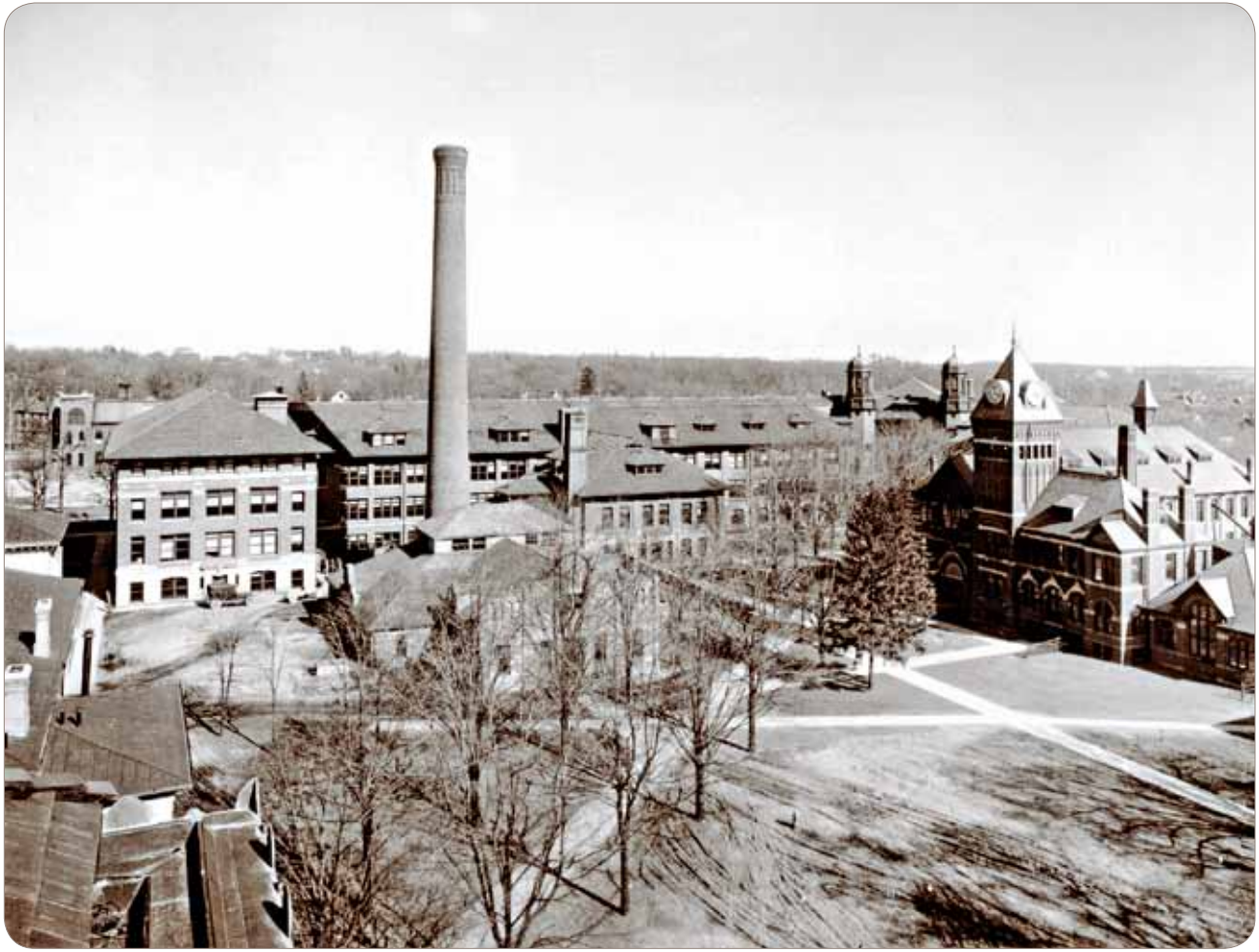
Engineering - Central Campus - circa 1920s
