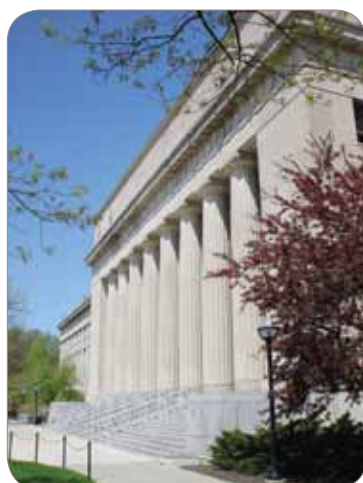
Angell Hall Renovation
