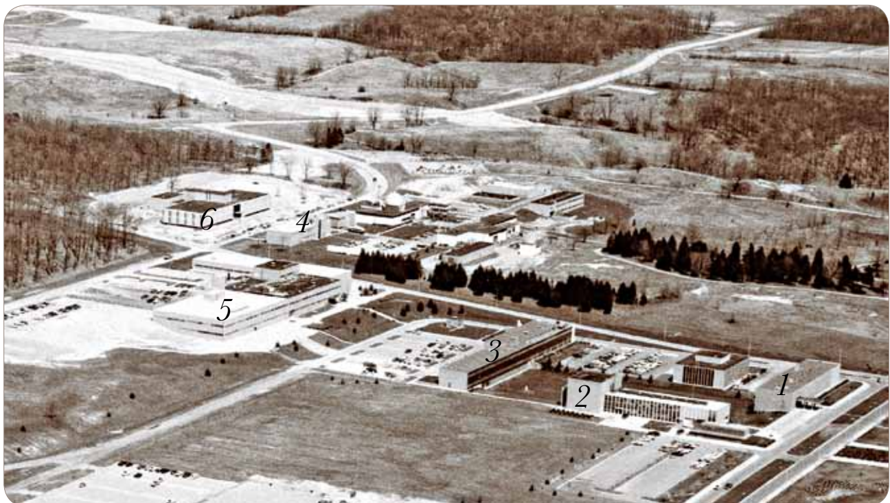
Engineering Buildings on the North Campus before 1970
