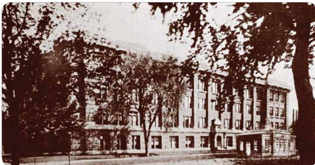
The New Chemistry and Pharmacy Building (The original Chemical Laboratory is inset at lower right.)
