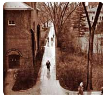
Physics Laboratory Addition (left)
