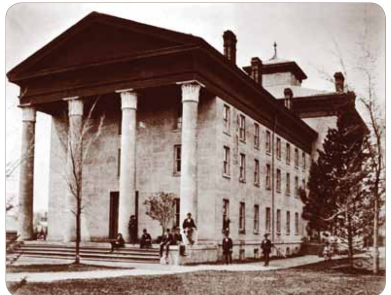
Original Medical Building
