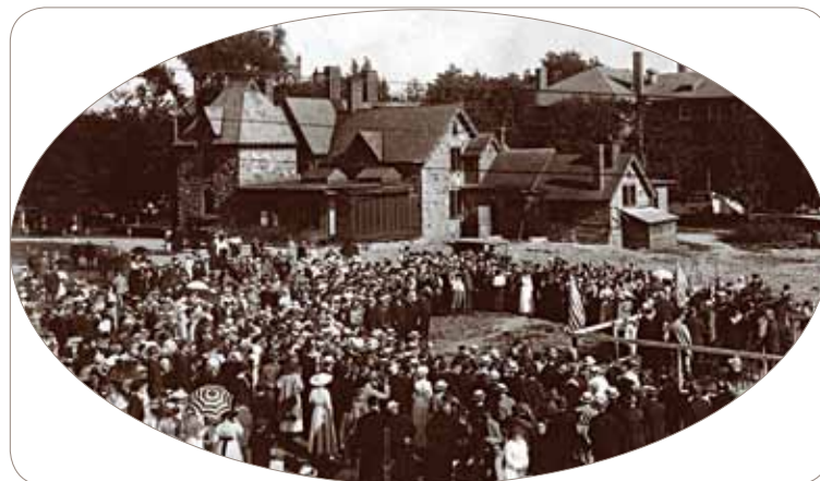
Groundbreaking for the New Michigan Union
