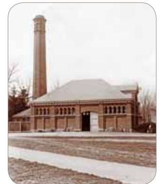
Heating Plant Behind University Hall
