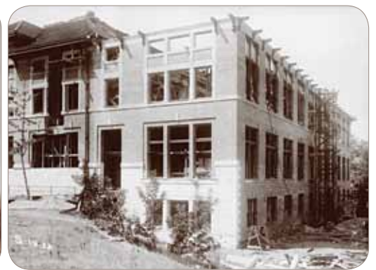
Dental Building Addition 1923
