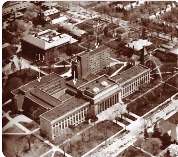
Mason Hall (1) Auditoriums (2) Haven Hall (3)
