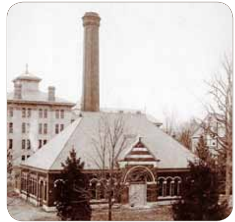
Heating Plant - Medical Building (rear)
