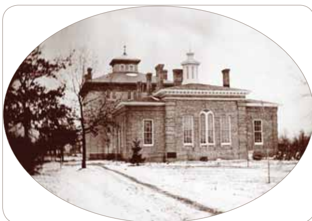
Chemical Laboratory 1864 Addition to the Medical Building (rear)
