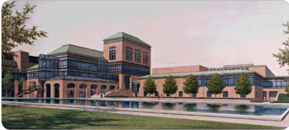
The Lurie Engineering Center
