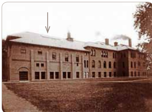
Physics Laboratory Addition (left)
