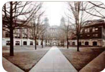
New Engineering Building
