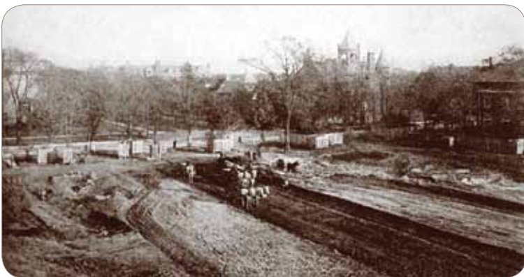
Excavation for the New Michigan Union
