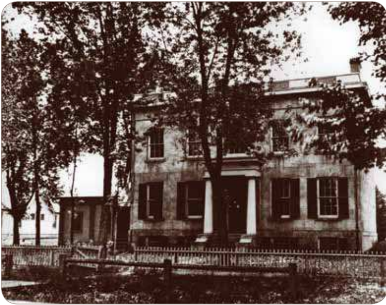
Original Professors' House (facing street)
