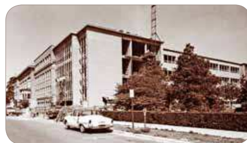
Frieze Building Addition 1957
