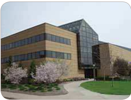
The FXB Building
