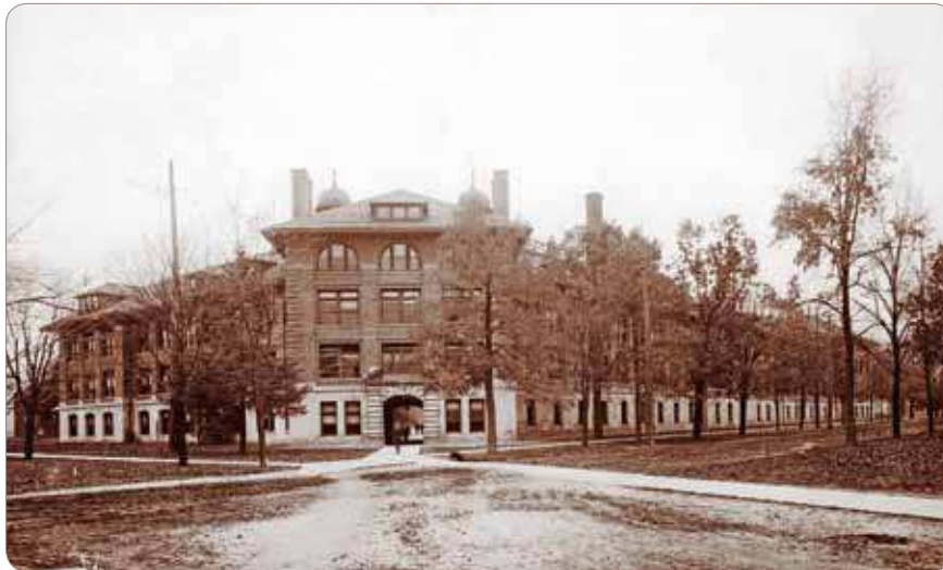
The New Engineering Building
