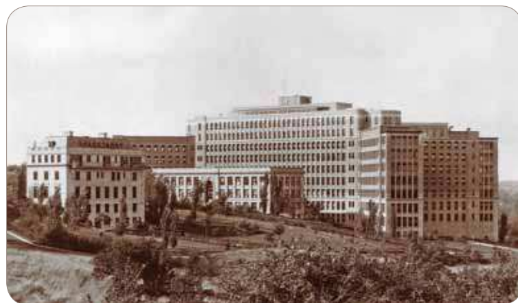
University Hospital with Two-Story Addition - Simpson Institute (left)
