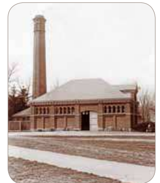
Heating Plant Behind University Hall
