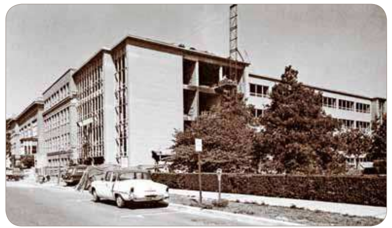
Frieze Building Addition 1957
