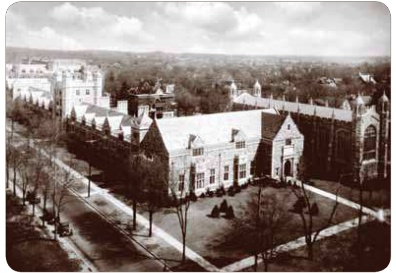
Dormitory Wing, Lawyers Club and Dining Hall
