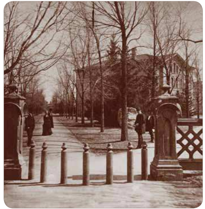
Fence with Posts
