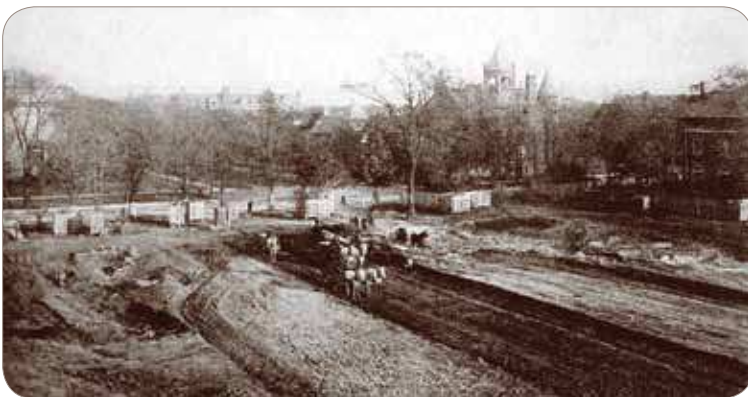
Excavation for the New Michigan Union
