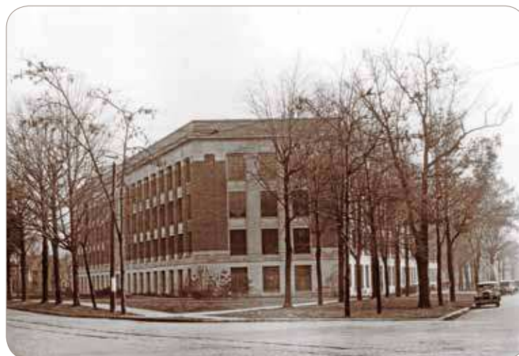
East Medical Building
