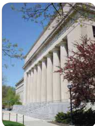
Angell Hall Renovation
