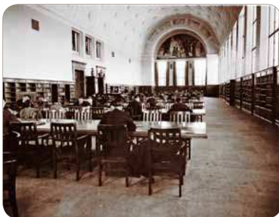
The General Library Reading Room 1920 (Melcher's Lunettes moved from University Hall)
