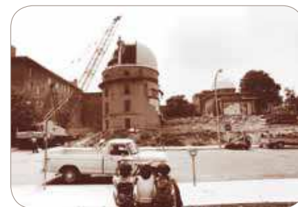
Demolition of the old Astronomy Building
