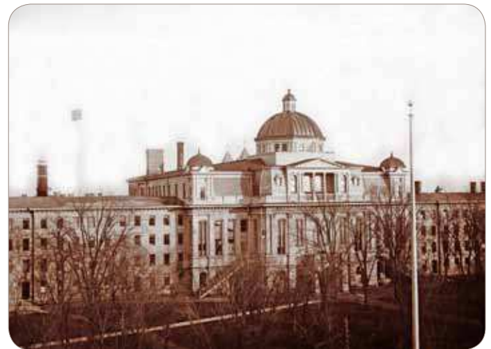
University Hall with Short Dome and Balustrades Removed
