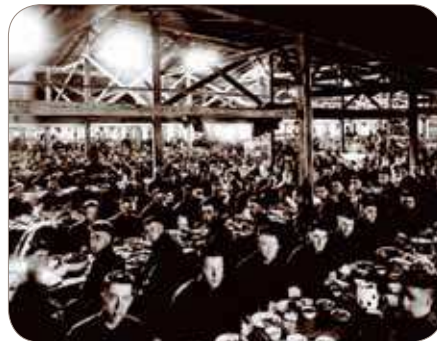
Temporary Mess Beside the Michigan Union
