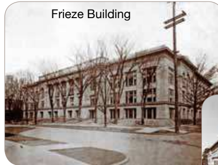
Frieze Building Addition
