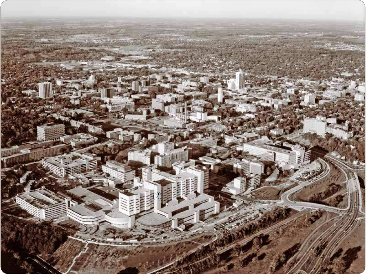
Old Main Hospital (1) Replacement Hospital (2)
