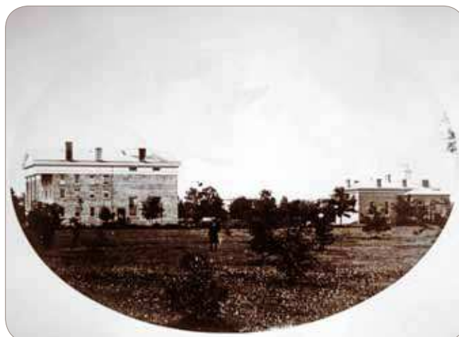
Medical Building (left), Chemical Laboratory (right)
