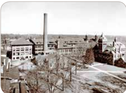
West Engineering, Engineering Shops Old Heating Plant
