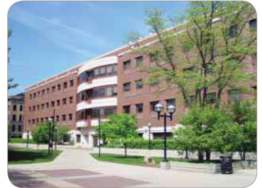
Randall Physics Addition
