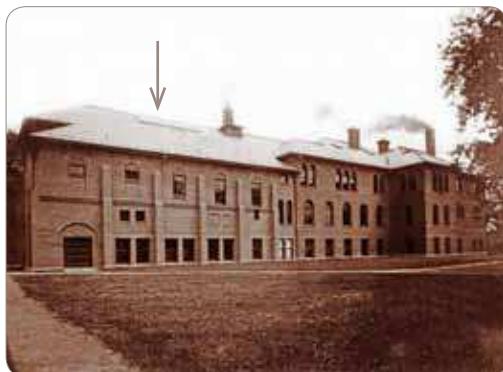
Physics Laboratory Addition (left)
