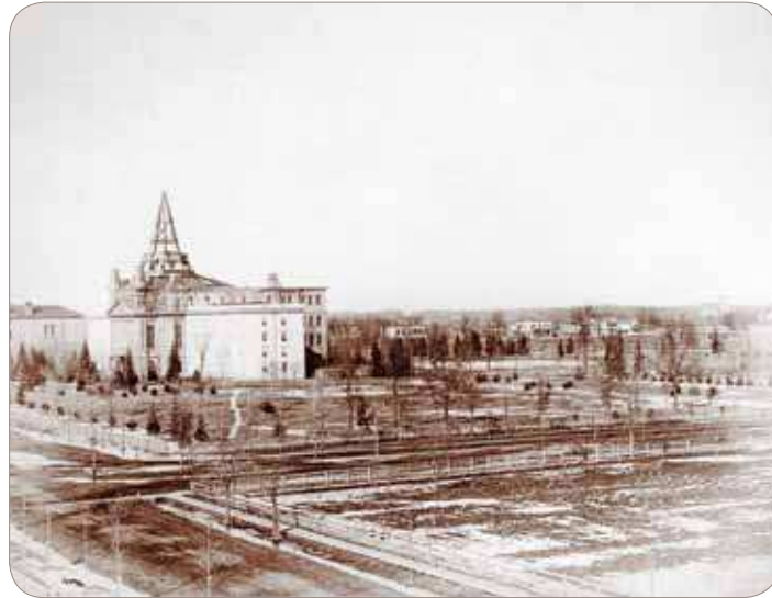
University Hall under Construction Completed in 1872
