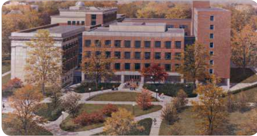
Tisch Hall - Angell/Haven Addition
