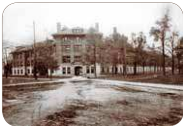
New Engineering Building
