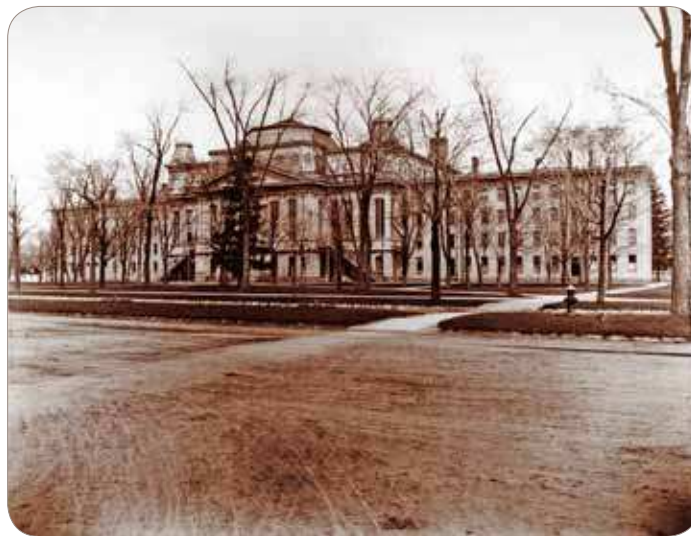
University Hall After the Tall Dome Had Been Removed
