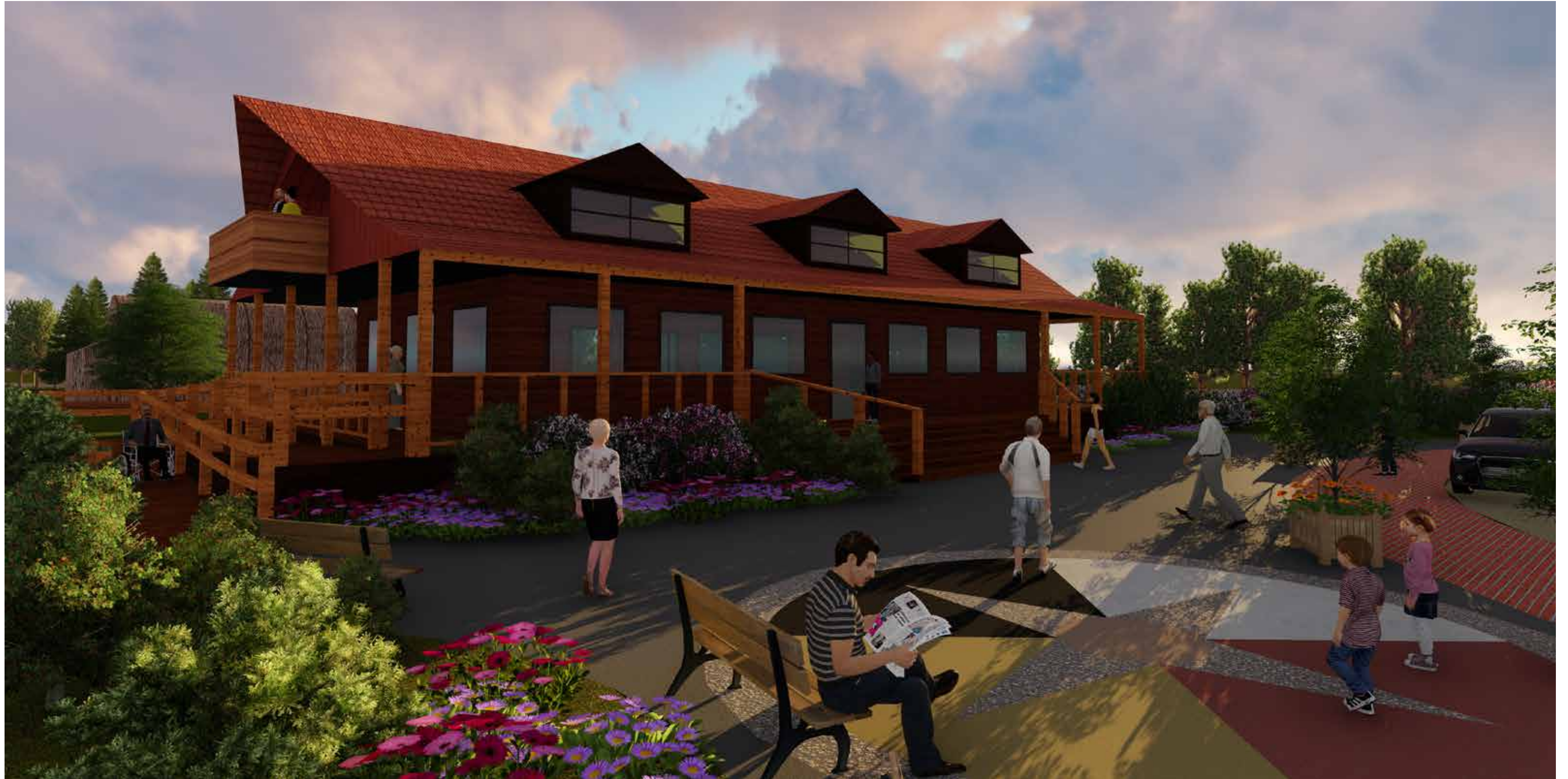
20 Main plaza before museum. This space welcomes visitors to Six Points and immediately immerses them into Wyandot culture.
