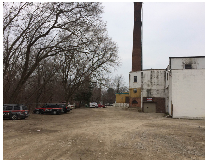
Existing lot behind the Historic Winery building
