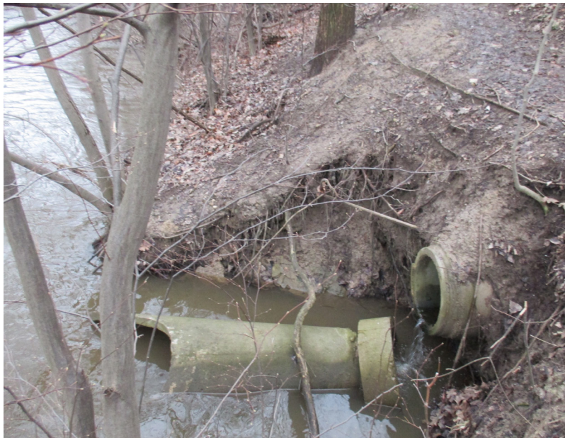
Stormwater outfall that empties directly into the Rouge River
