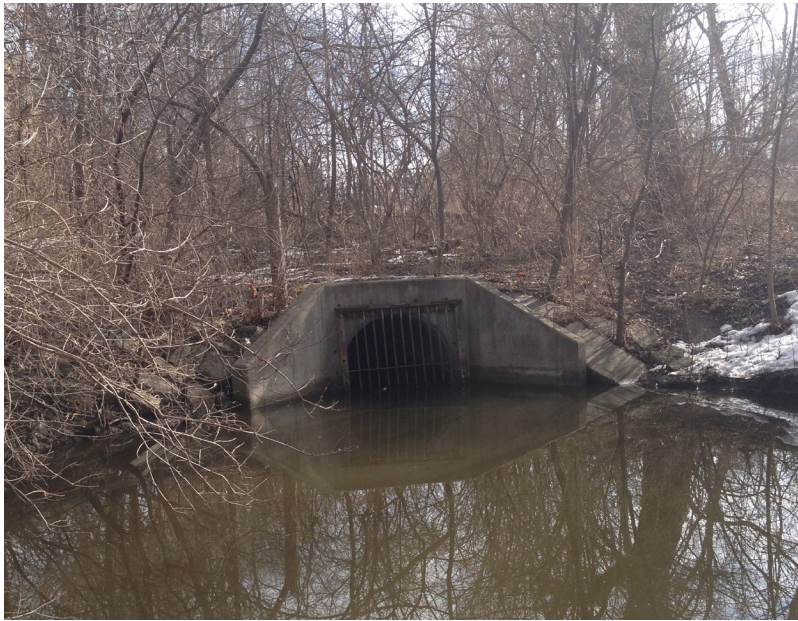
Stream channelization under 9 Mile Road
